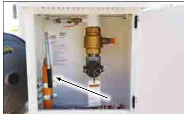
Fig 21 - Hand pump inside fill box
