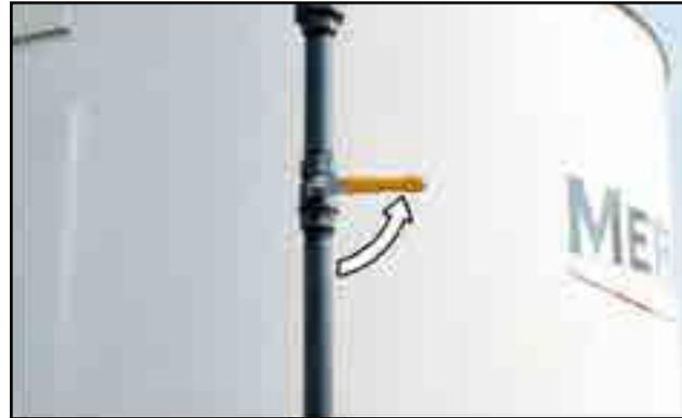
Fig 27 - Close shut-off ball valve
