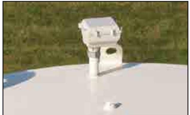
Fig 11 - Tank level gauge
