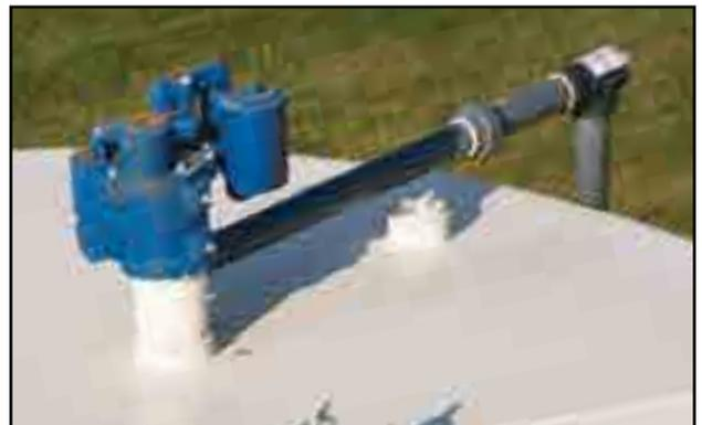
Fig 13 - Top-mounted fuel pump
