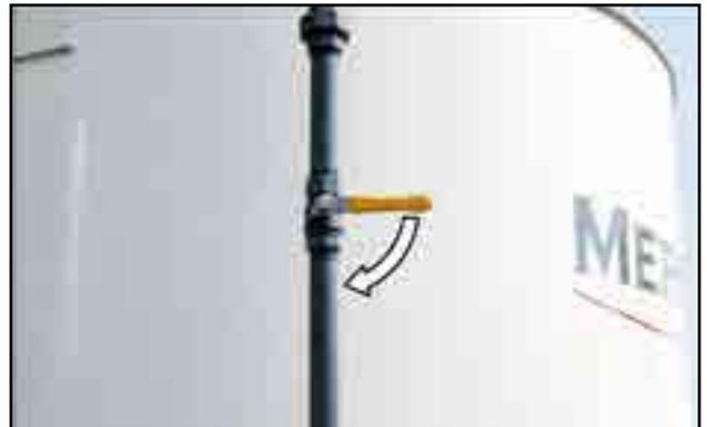
Fig 23 - Open shut-off ball valve
